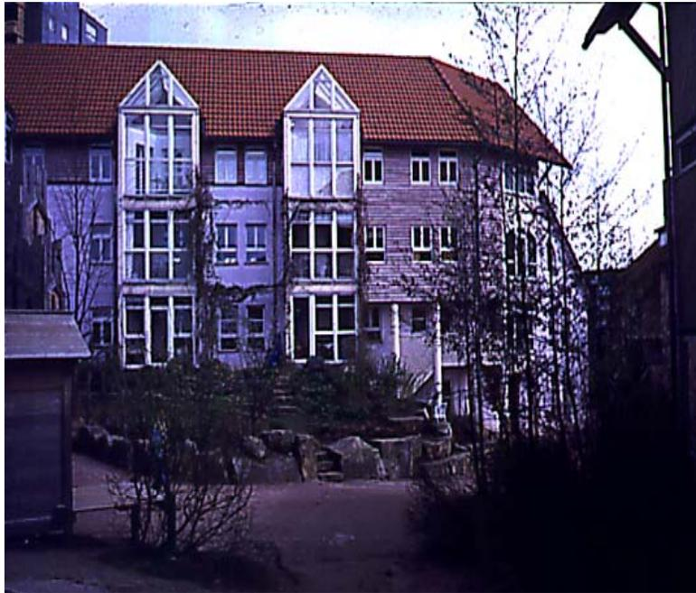
The form of the buildings became ever more related to passive solar gain and a preference for large south and small north facing windows. Phase 7 formed a sun-scoop using a permaculture garden design. The extent of landscaping is rich and varied, and allows for larger areas of soft and porous surfacing. The next phase under development contains low allergy materials and finishes. The ventilation will use dynamic insulation.
