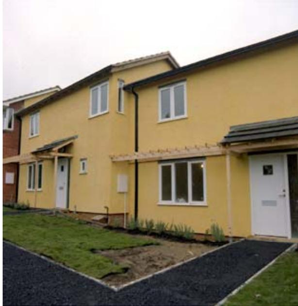
A French company, Isochanvre ([www.isochanvre.com](http://www.isochanvre.com)) have developed, in partnership with Suffolk Housing Society and Modece Architects, two prototype hemp/lime houses in Suffolk which have been monitored by BRE against two otherwise identical conventional houses.
